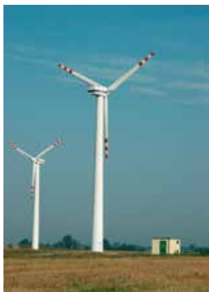
wind farm Windpark
