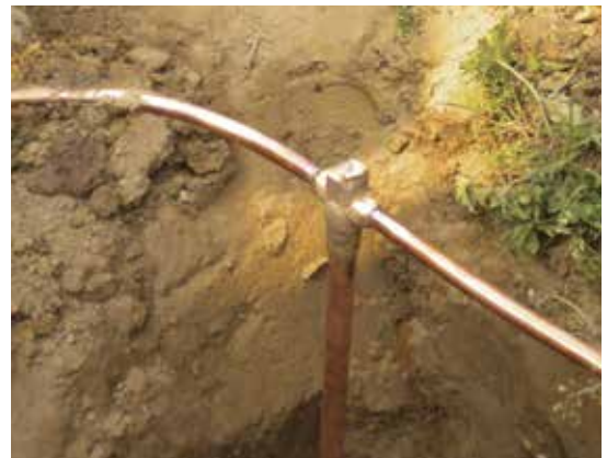
GT Cadweld connection
