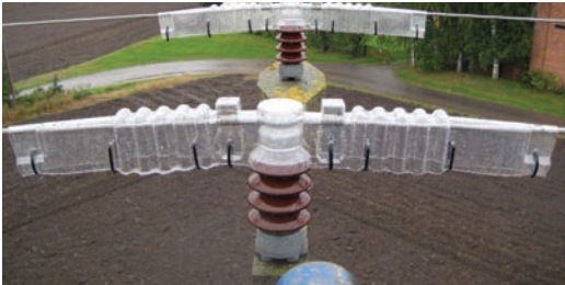
BCIC-1217-TR: Post Insulator application
