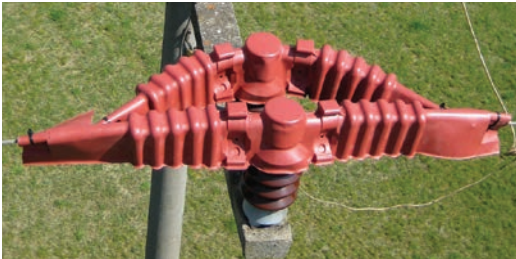
BCIC-1215: Double Post Insulator application
