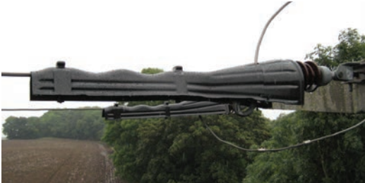
BCIC-TEN-01: Tension Insulator application
